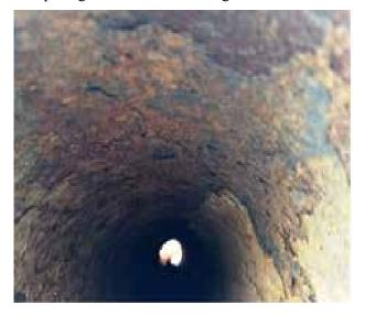
Fig. 1. Corroded 300 mm Dia Fire Fighting Pipe Line
